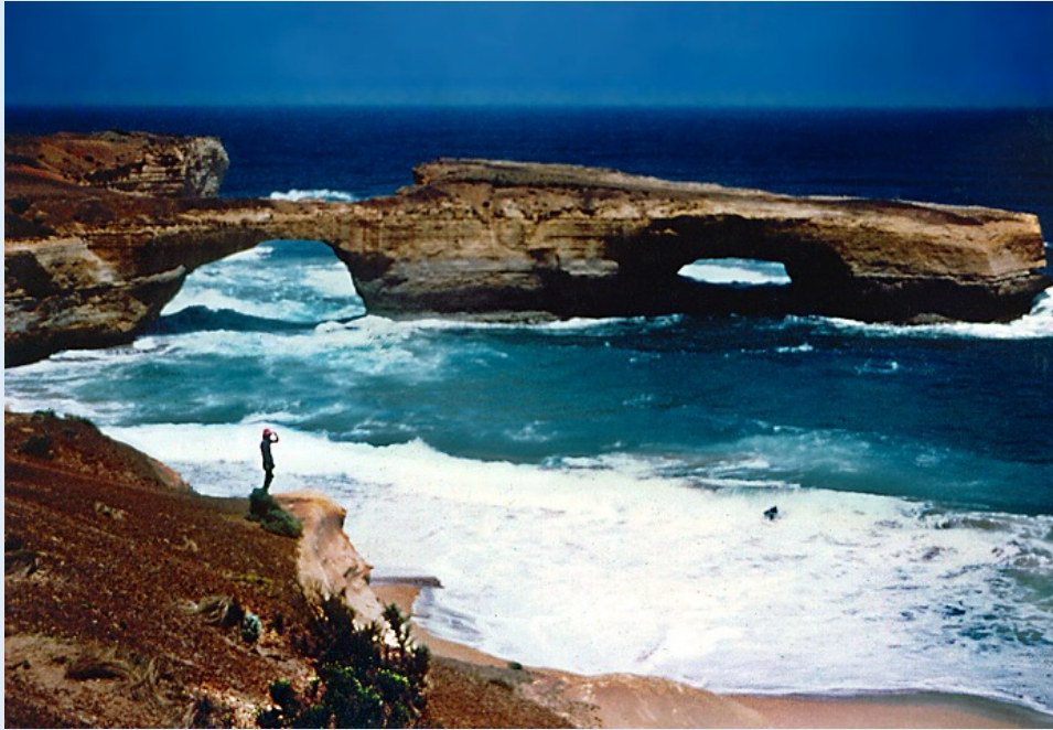
London Bridge Port Campbell prior to collapsing in 1990
